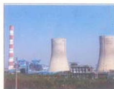
Asia's largest Cooling Tower & Chimney, Simhadri STPP (AP)
