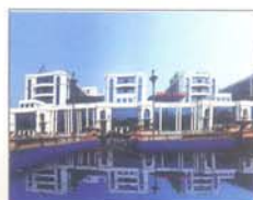
NBCC Plaza, Pushp Vihar, Saket, New Delhi - Real Estate Project
